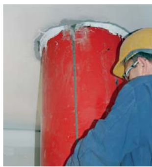
Pumping concrete from the base to ensure a high quality surface finish
