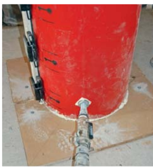
Pumping concrete from the base to ensure a high quality surface finish
