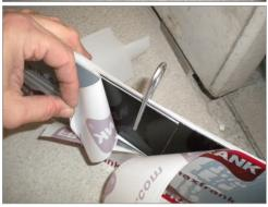
Only remove the upper protective film tape prior to installation of the reinforcement and / or before closing the formwork.
