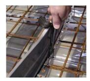
B) Fradiflex metal water stop with fixing angle
