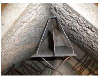
Due to the considerable inherent stability of Fradiflex metal water stops they do not need to be fixed to the element wall.
