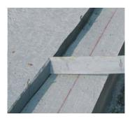
Only remove the upper protective film tape prior to installation of the reinforcement and / or before closing the formwork.
