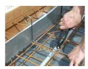
A) Fradiflex metal water stop without fixing angle
