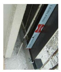
Position metal water stop so that it will be integrated into the element wall's controlled cracks up to the half width each.
