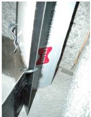
The erected and fixed metal water stop for element wall's controlled crack joint flashing is then simply built against the element wall.
