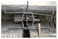
Shortly before concreting the metal water stops for element wall's controlled crack joint flashing are fixed with special, re-usable fixing loops. Different types of fixing loops are required for joints and corners; different wall thicknesses require different dimensions of fixing loops as well.
