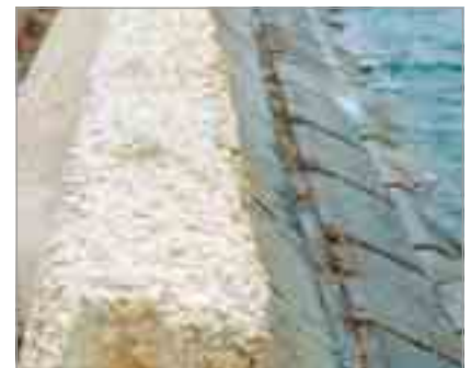
Concrete surface degraded by sea water
